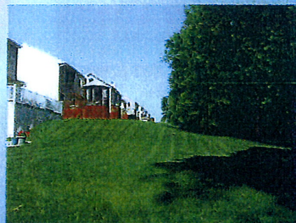
Disconnection of Rooftop Runoff
